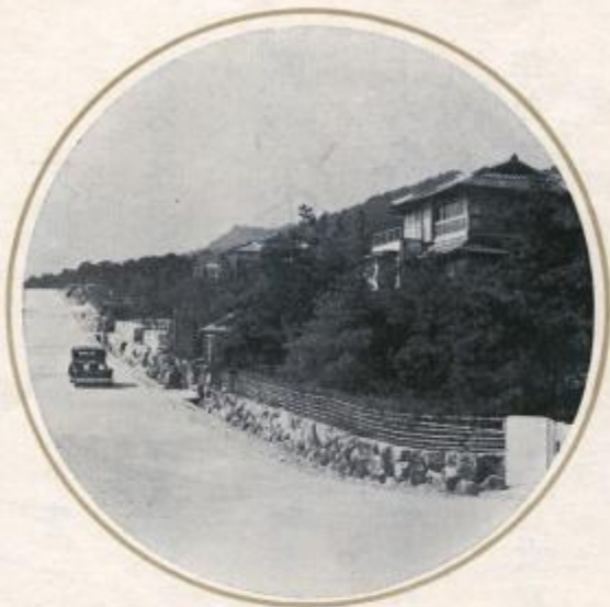
通橋合落部一ノ路道内莊
